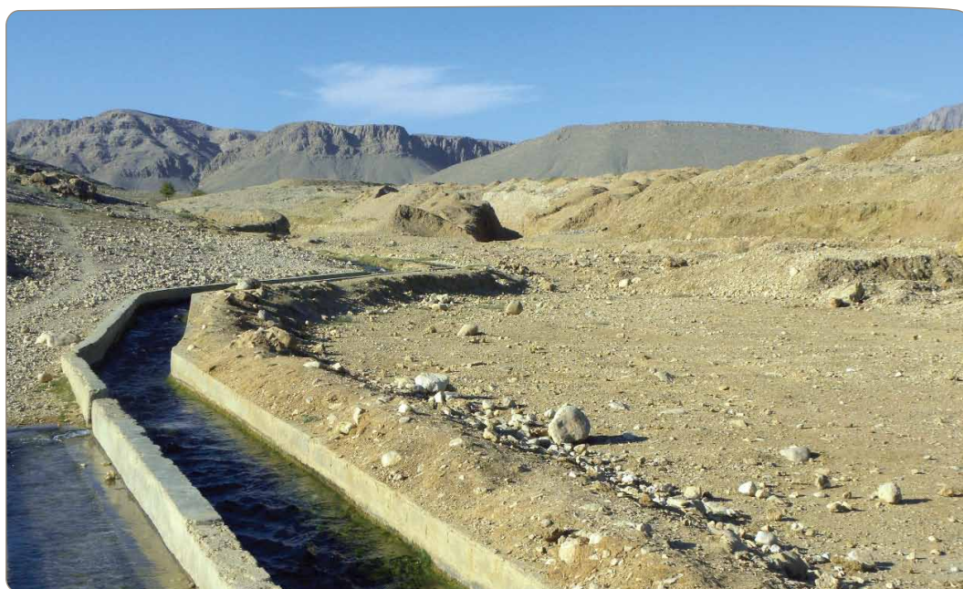
Lining of Karez s helps considerably in minimizing conveyance losses associated with surface water flows
