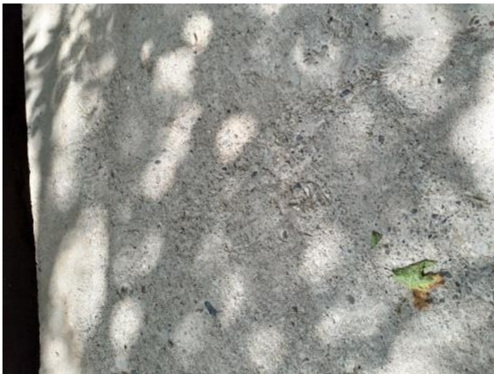
Erosion of Concrete due to PCC 1:3:6 at Link Road Tauheedabad
