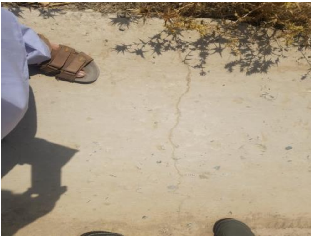
Cracks Observed at Bahrampur Link Road
