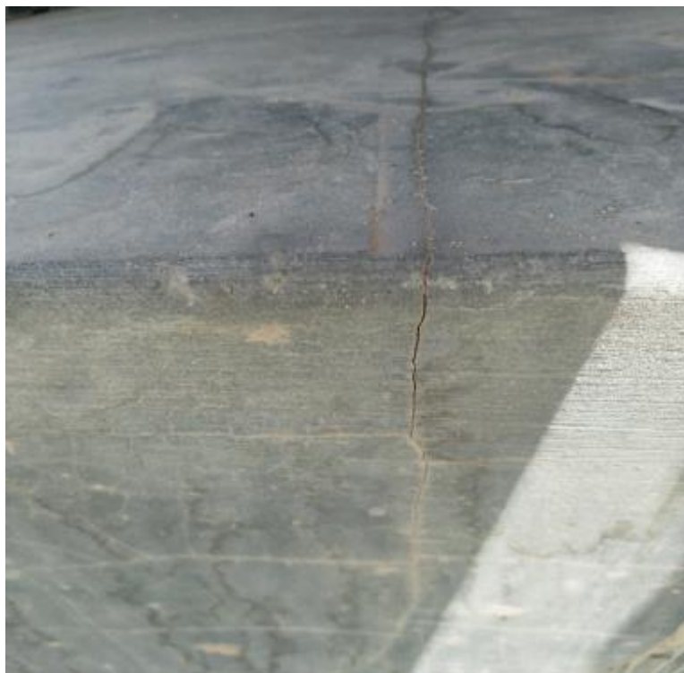
Cracks Developed in Water Pond due to Soil Pressure
