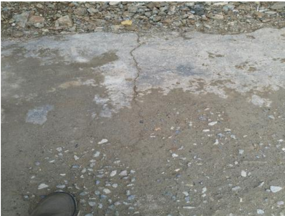
Erosion of PCC due Heavy Load and Cracks due to Long PCC Panles
