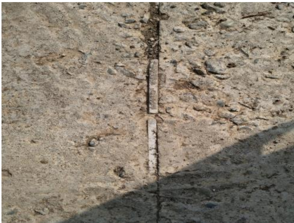
Marble Strips as Flexible Joints Cracked due to its Rigidity
