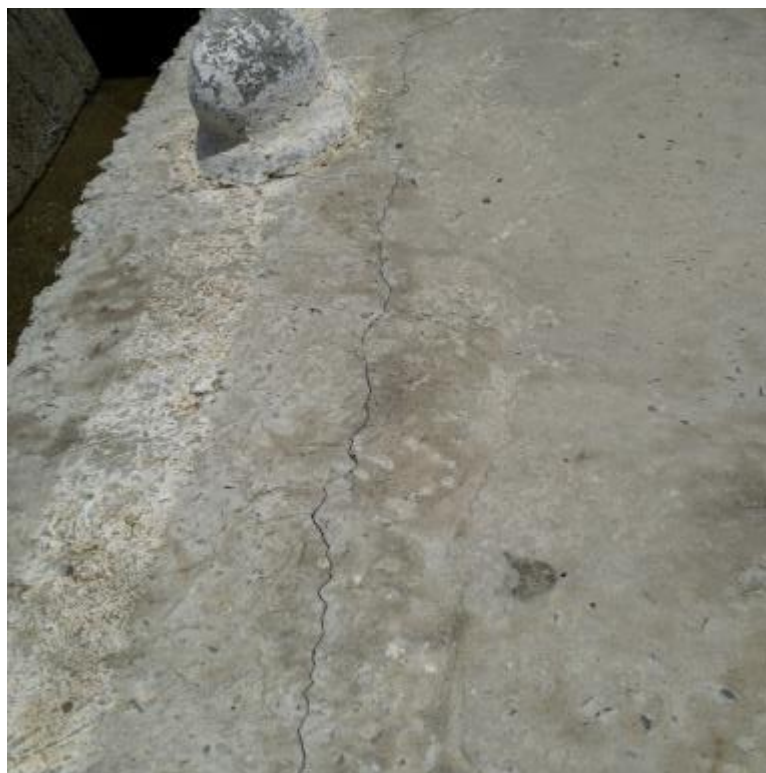
Major Cracks and Erosion of PCC due to Improper Load Calculation of Traffic and Long Panels more than 20 ft
