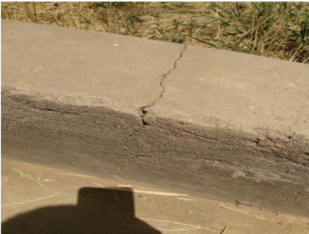
Minor Cracks Developed in Wall of Channel
