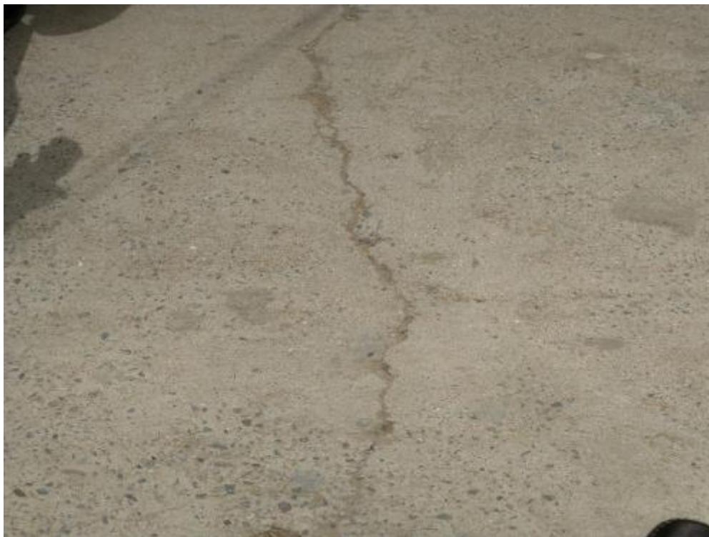
Major Cracks and Erosion of PCC due to Improper Load Calculation of Traffic and No Panels
