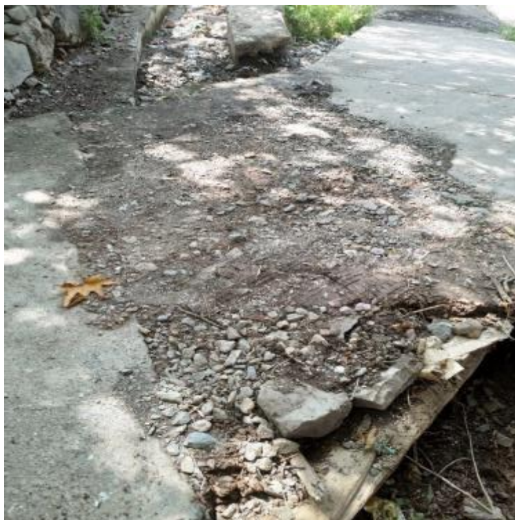
Pipe Culvert Missing at Tauheedabad Link Road
