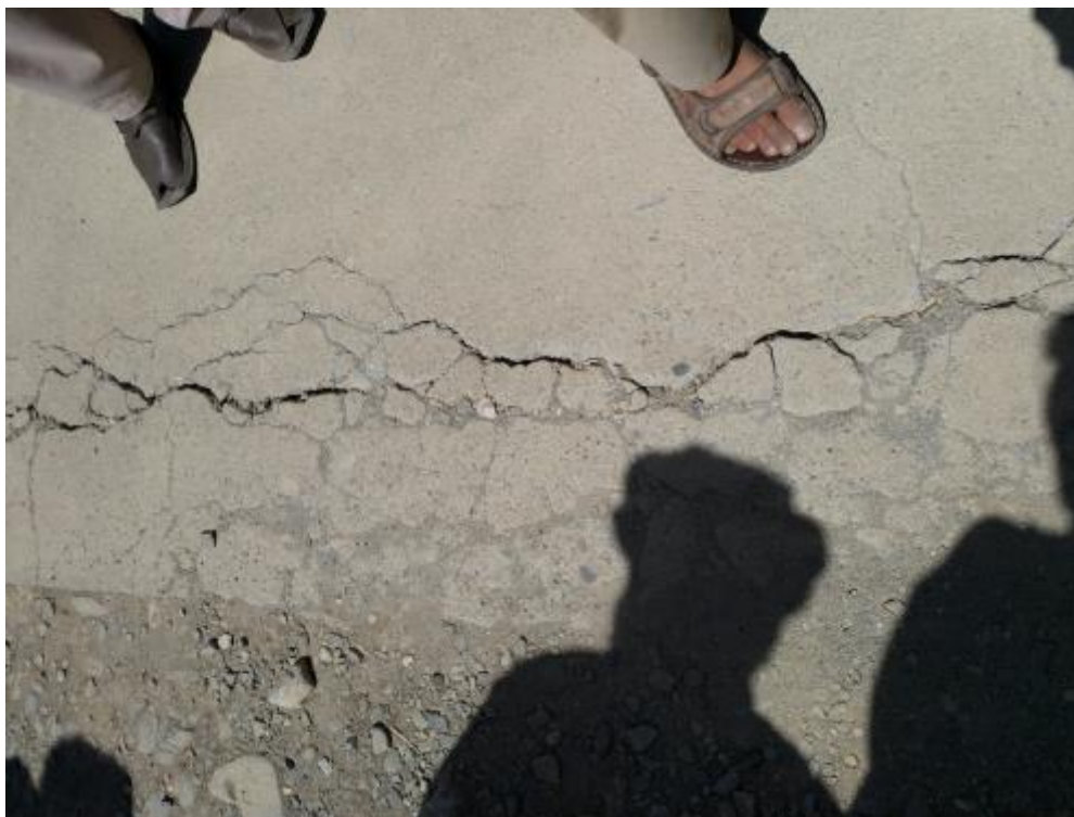
Major Cracks and Settlement of Link Road at Potoniandeh due to PCC 1:3:6
