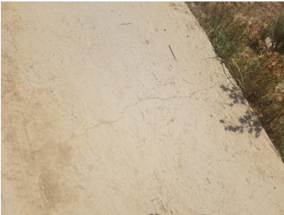
Cracks Observed Koka Link Road
