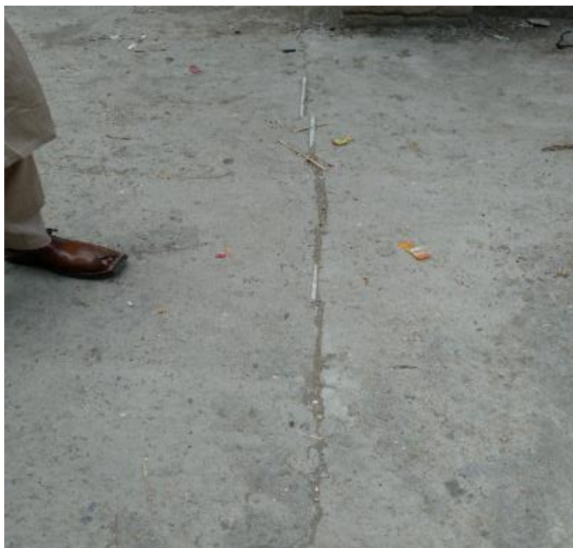
Marble Strips as Flexible Joints Cracked due to its Rgidity
