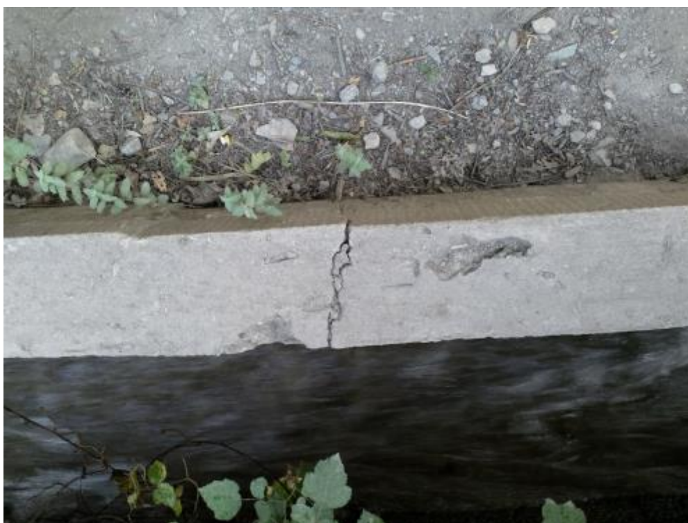
Major Cracks Due to PCC 1:3:6 at Irrigation Channel Broon
