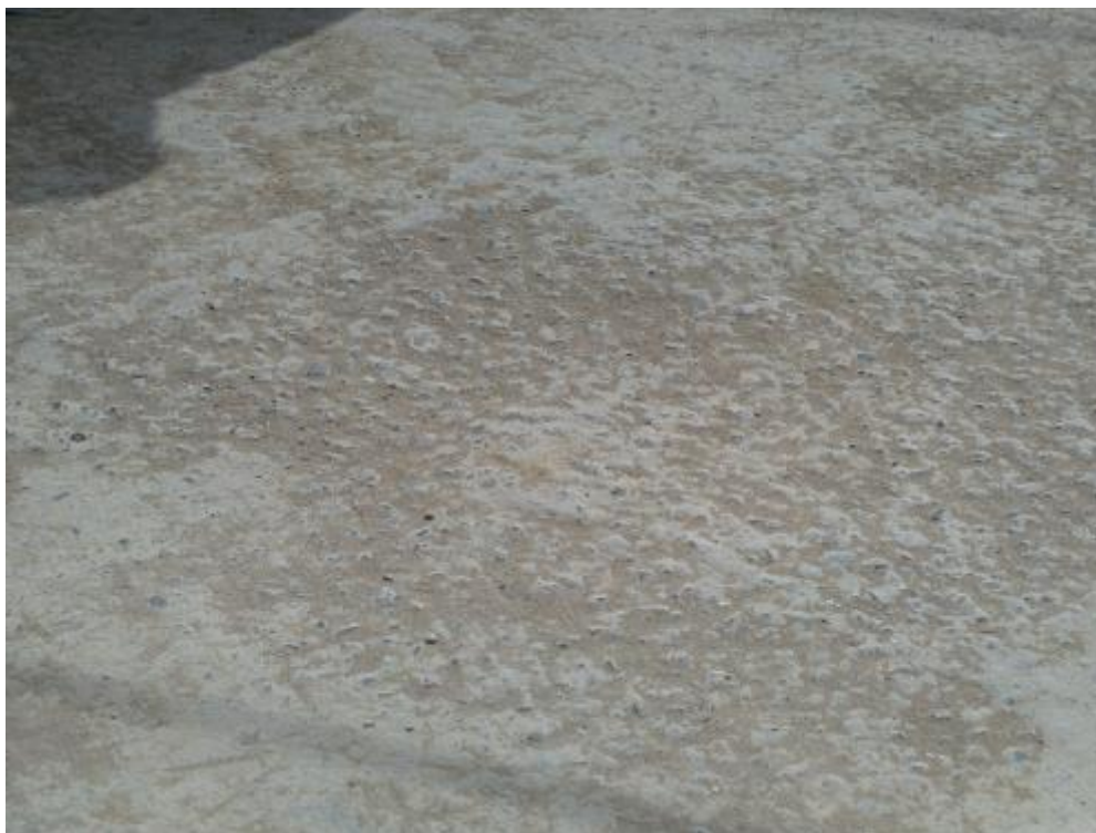
Erosion of PCC due to Improper Load Calculation of Traffic
