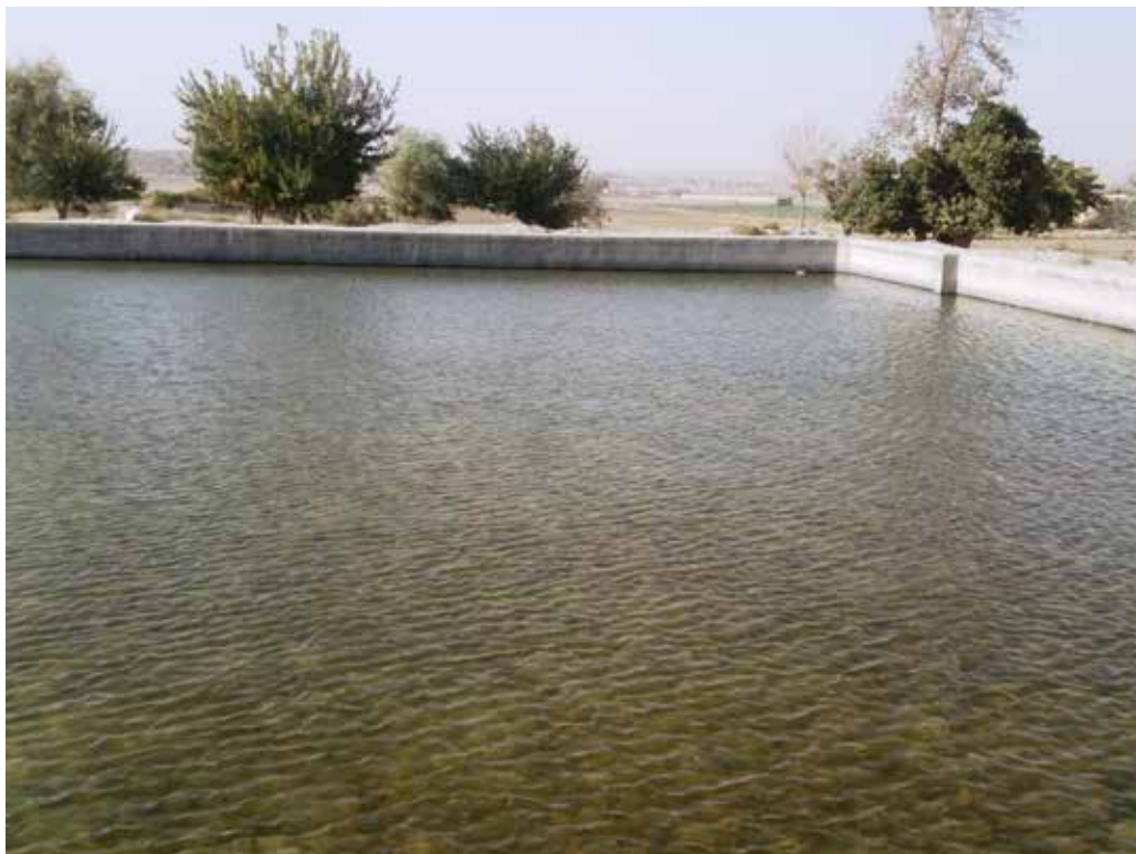
Water Storage Reservoir - Pishin
