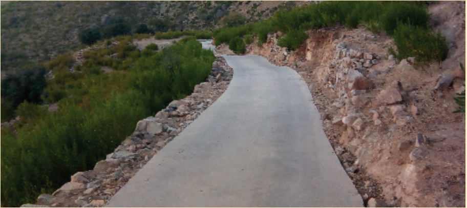
Link road improving access to Village Hisarak Payeen after the construction
