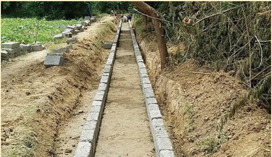
The under construction irrigation canal in Haji Khandero Goth in Sakran
