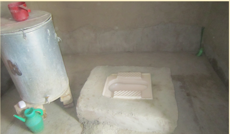
Low cost laterin built to discourage open defecation practice
