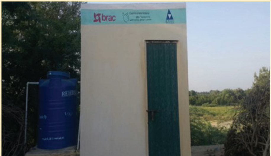
A latrine build to make Sabz Ali Goth Open Defecation Free (ODF) village
