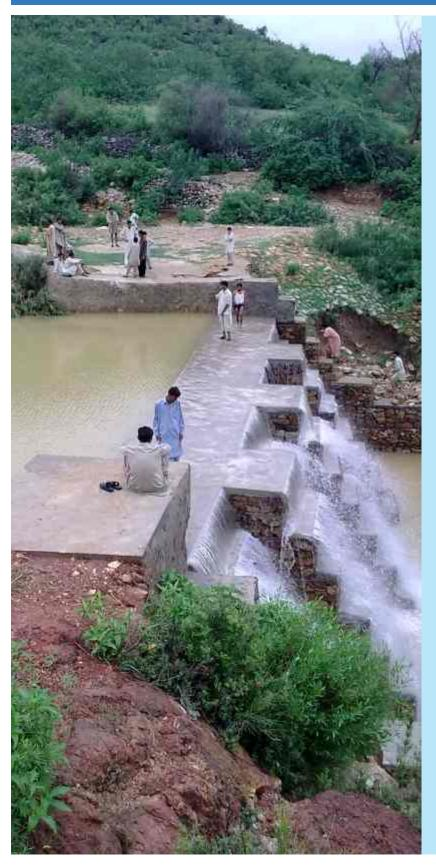
PPAF initiated Drought Mitigation and Preparedness Program (DMPP) to mitigate severe drought conditions in some of the most adversely affected parts of the country. The DMPP typically includes construction of delay action/check dams for improving underground water table in addition to meeting the community's domestic and agricultural requirements. These delay action/check dams have also served as a great protective measure for saving the communities from recent flood waters.
