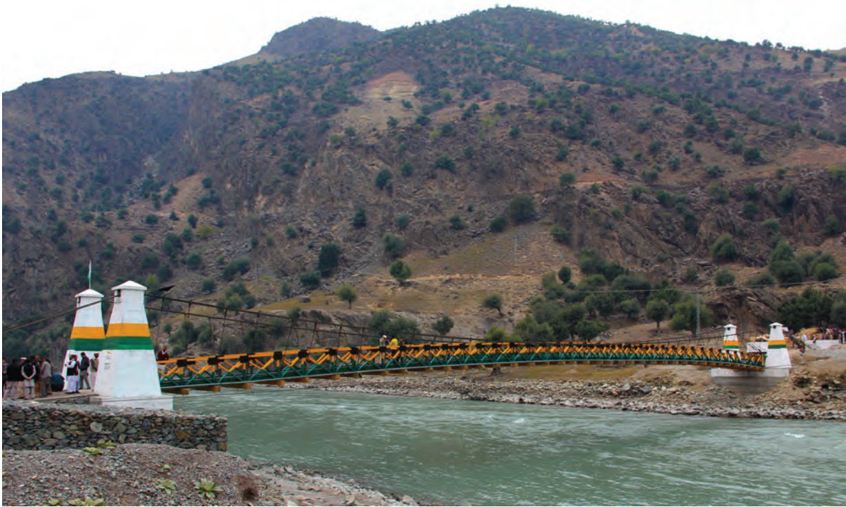
Suspension Bridge built under PPAF's LACIP initiative at Ashraits, Chitral, KP
