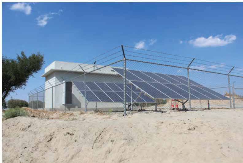
PPAF's solar mini grid project at Motara Korona, Lakki Marwat, KP
